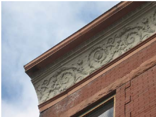
Sheet metal cornice at 429 N. Roane Street (above); cast iron pilaster at 420 N. Roane Street (right).
