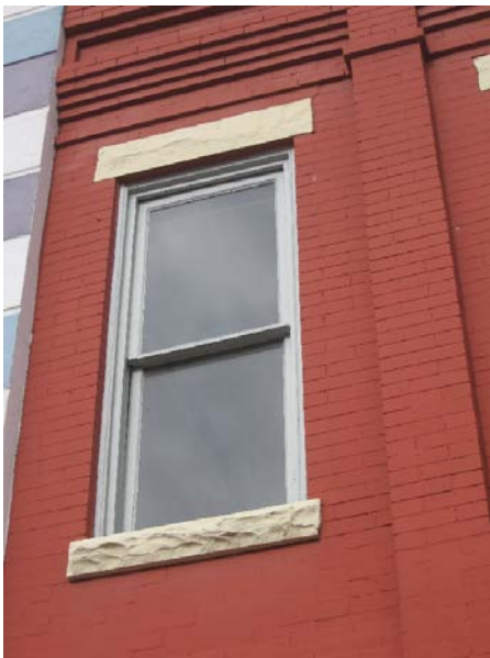
Original one-over-one wood sash windows at 423 (left) and 428 (right) N. Roane Street
