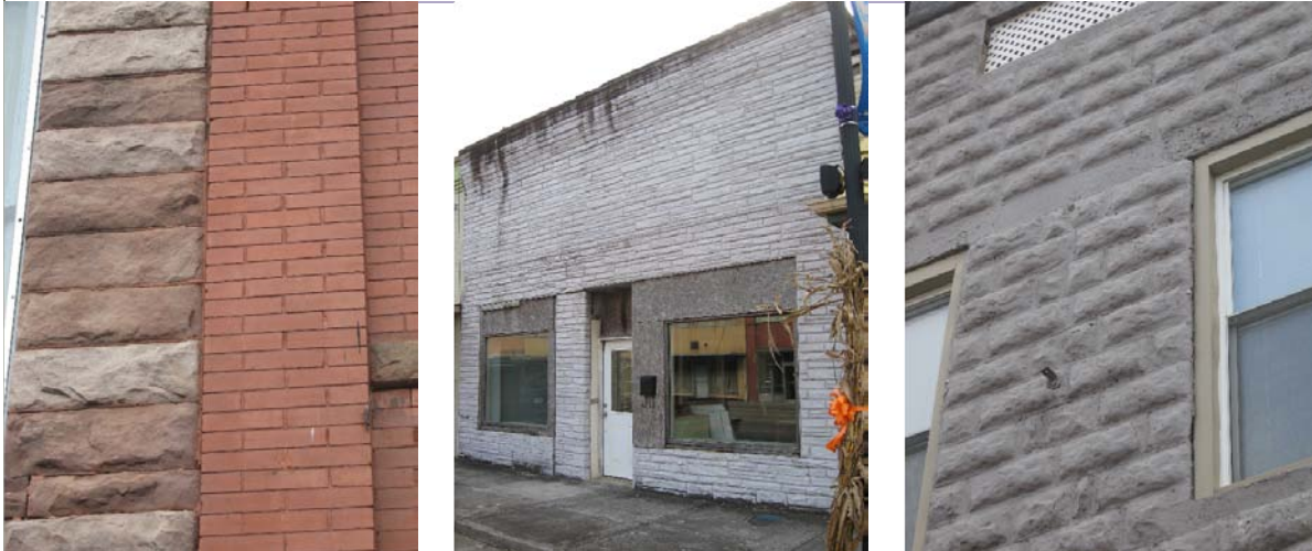
Stone and brick masonry at 413-415 N. Roane Street (left); formstone exterior at 518 N. Roane Street (center); rock-faced concrete block at 426 N. Roane Street (right).
