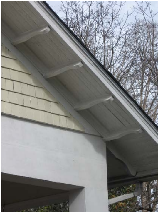
Preserve original roof features such as eave brackets and exposed rafter tails (429 Cumberland Street).
