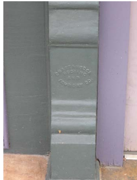
Sheet metal cornice at 429 N. Roane Street (above); cast iron pilaster at 420 N. Roane Street (right).
