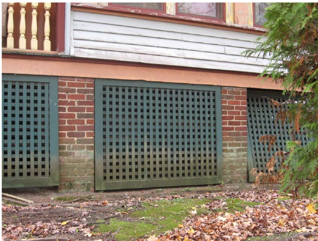
This dwelling has appropriately designed and placed lattice panels in the porch foundation (530 Clinton Street).
