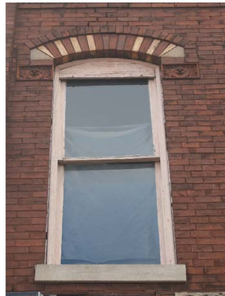
Original one-over-one wood sash windows at 423 (left) and 428 (right) N. Roane Street
